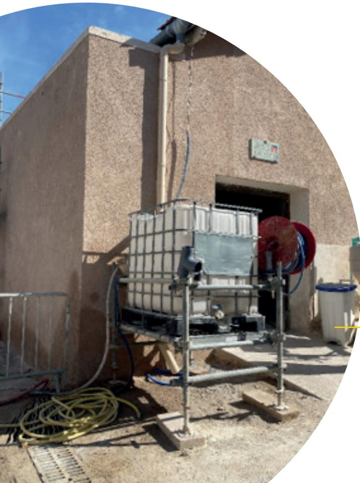
*Example of a water tank collecting rainwaters for cleaning tolls
